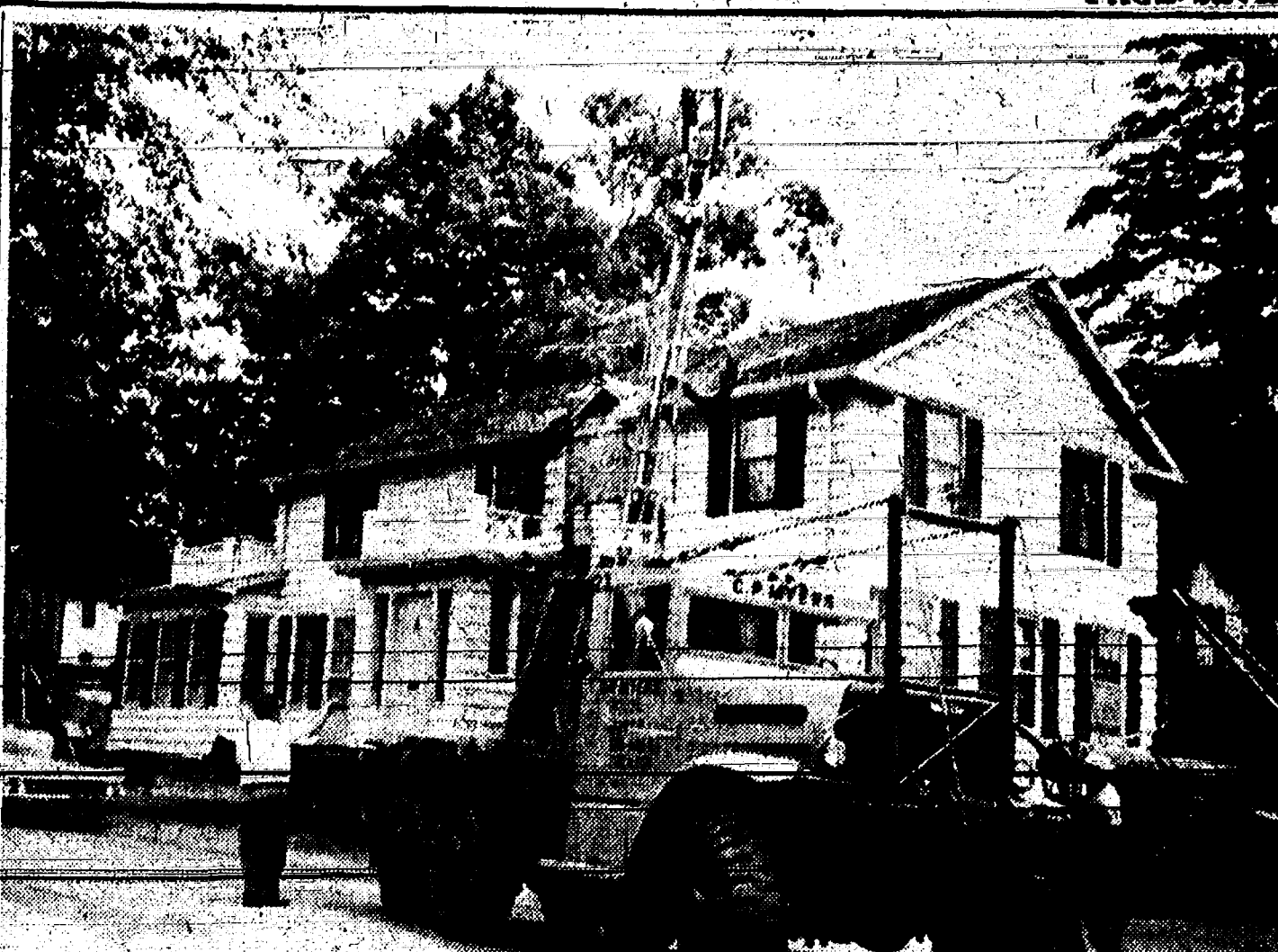
SEEING THINGS? This house, slowly meandering down Chelsea's Main St., was not an optical illusion — it was the residence of Mr. and Mrs. George Palmer. The structure, a four-bedroom home which has stood at its 221 S. Main St. location for over 100 years, has been moved to make room for a parking lot at Palmer Motor Sales. Preparation for the move took five months almost a week, and the move itself started at 9 a.m. Monday morning, was not completed until 11 p.m. The movers, C. P. Myers of Trenton, moved at a snail's pace down Main St., then onto Old US-12 to the new location north on Freer Rd. The route was selected because there were fewer turns, low hanging limbs and wires to be moved. The house is shown near Van Buren St. as the contractors lifted telephone wires to allow the house to pass beneath. None of the furniture was removed from the house for the move.
